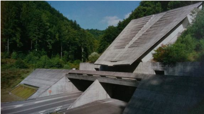
Image taken from The Landscape of Contemporary Infrastructure / 'Tunnel Artifice' (1988-2008) by Architects Renato Salvi and Flora Rucjat-Roncati / on page 146-147
